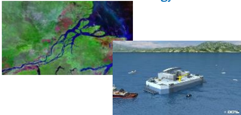
Ocean Thermal Energy Conversion
